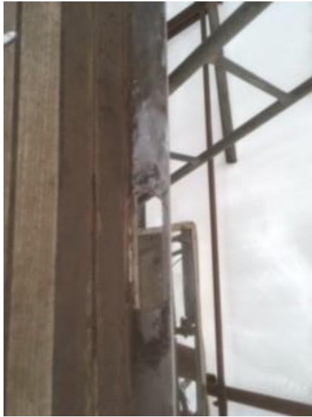
The teak on the inner and outer side of the capping rail came off and the corrosion was treated properly with sandblasting and corroless paint.
